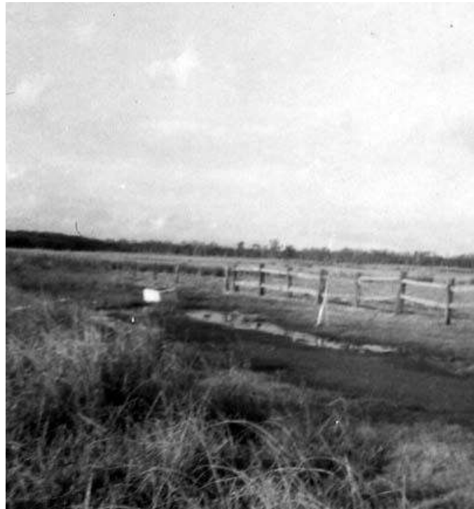
A-3 on pad with refrigerator shelter in background
